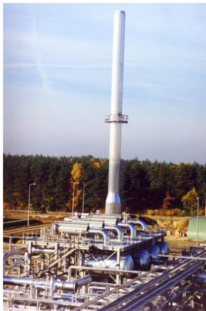
Sherritt Power Corporation – Boca de Jaruco, Cuba
